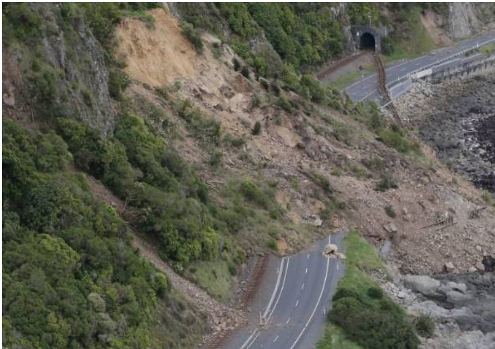
Figure 1: SH1 and the Rail Line Near Kaikoura (Source: Mitchell, 2016)
