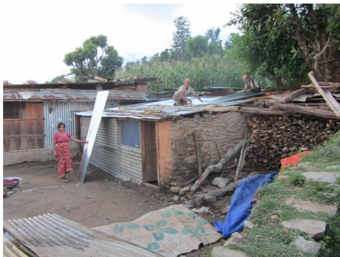
Figure 3. Villagers rebuilding their temporal shelter with CGI sheets
